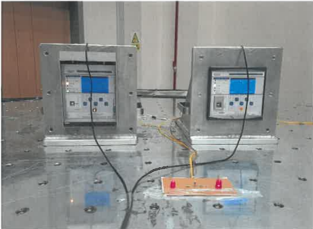
Picture 1. General View (Front)
